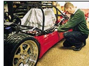
The first panels to be fitted are the sidepods. Using wheels for alignment, these house the fuel tanks and luggage containers. Once in position, sealant, pop rivets, and set screws locate the panel permanently.
