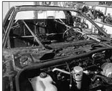
Temporary bracing was tack-welded across the cockpit and doors to keep the pan square after the roof is removed. Once the roof is removed, the chassis will warp, and it will be very difficult to get it aligned again. The roof will be removed with a Sawzall.
